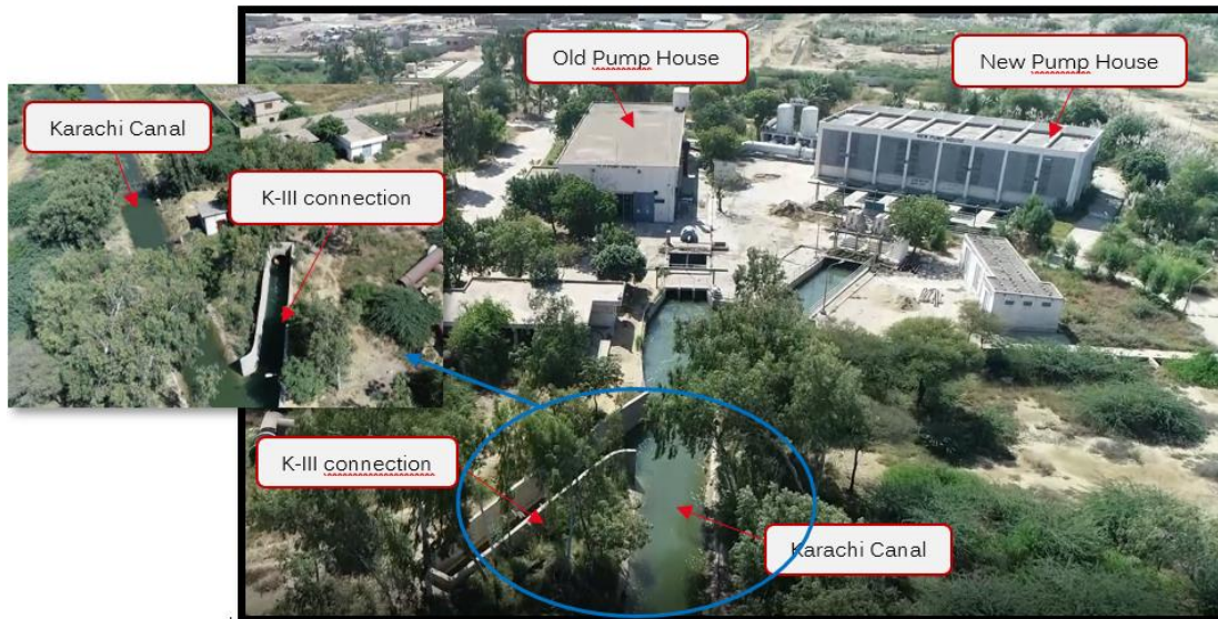
Figure 7: KWC, KIII Conduit, Old and New Pump Houses – Present Configuration.
