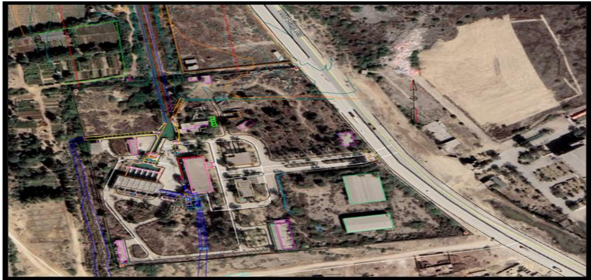
Figure 5: Access to the Pump Station from the Hub Dam Road.
